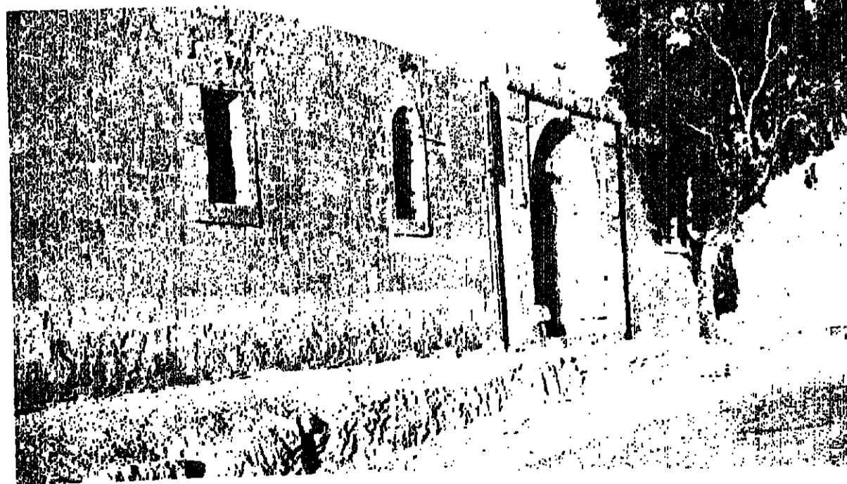
Inn building, which was used as a Turkish police post about the turn of the century.
